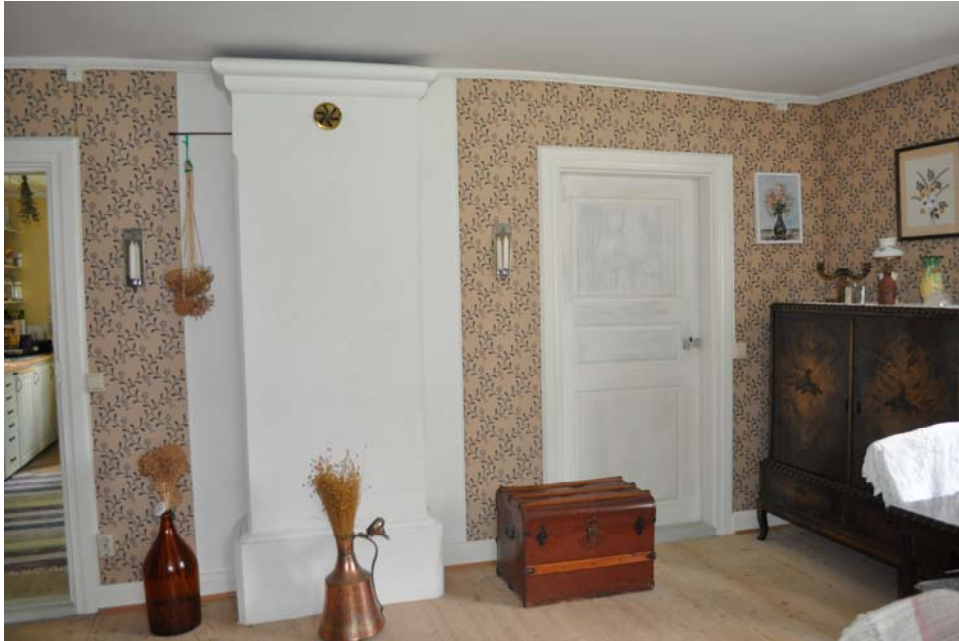
Livingroom with poor mans stove still in use. The flue gas from the kitchen stove is lead in channels inside the brickwork.
